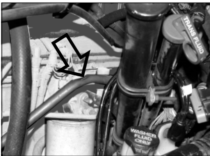
Damaged discharge line shown.
